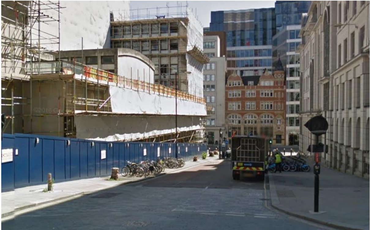
Stonecutter Street - before
